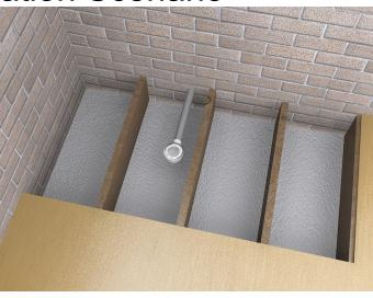
2. Now that the floor has been cut back, battons can be fitted. Note that the floor has been cut back so that it is resting half on the joist and can be screwed down.
