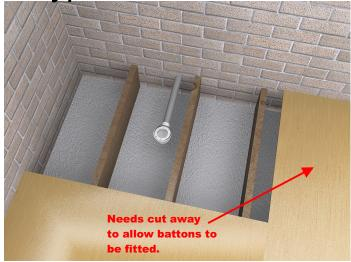
1. After cutting away the floor, areas that need to be supported with battons can be identified. In this case we can see that a further portion of the floor will need cut away to allow battons to be fitted.
