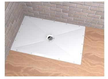
6. The floor former can now be screwed down to the subfloor along with the outer collar of the waste trap. A sheet of plyboard can be fitted to bring up the floor level flush to the floor former.
